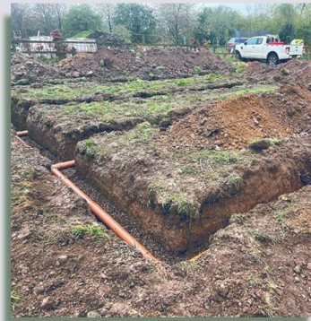
Drainage field designed to BS 6297 standard
