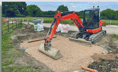
Reed Bed Installation
